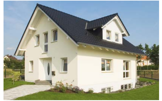
House Rügen II
